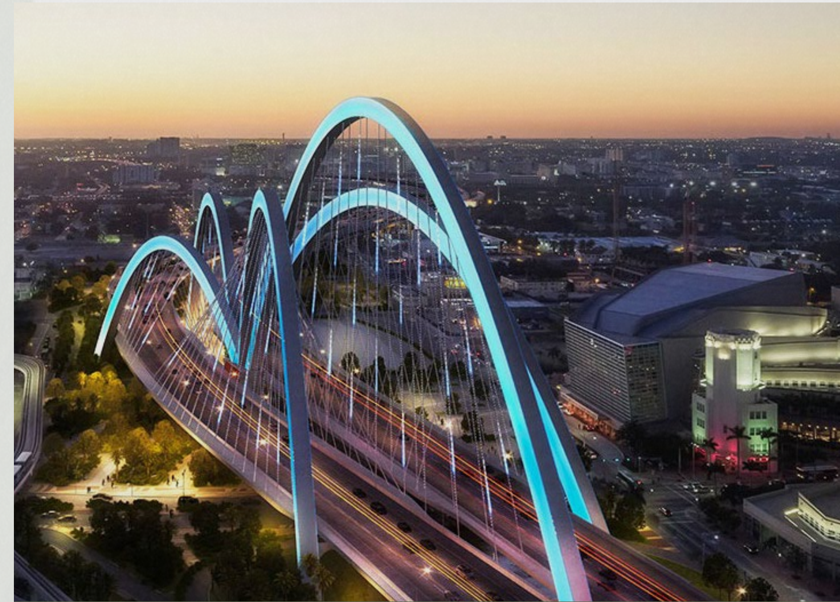
I-395 SIGNATURE BRIDGE
